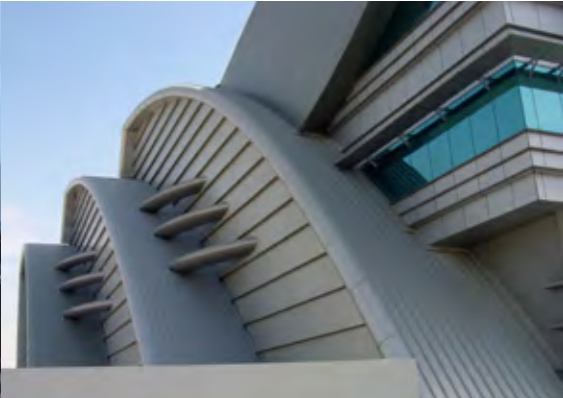
Dubai Flower Center // UAE Usage: retail Profile: N65 - 400 Material: 1.0 mm aluminum Color/Surface: silver metallic / PVDF Area: 13 000 m²
