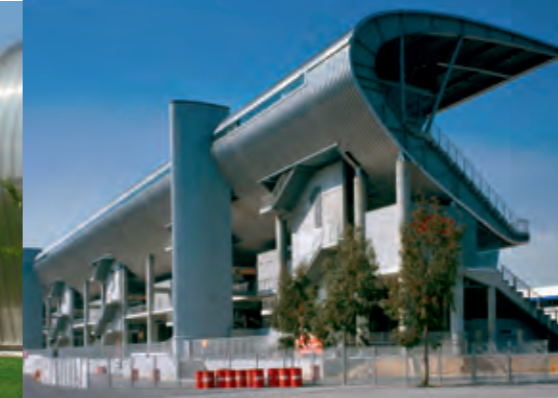
Formula 1 Grandstand // Spain Usage: sports Profile: N65 - 400 Material: 1.0 mm aluminum Color/Surface: bare aluminum Area: 17 000 m²
