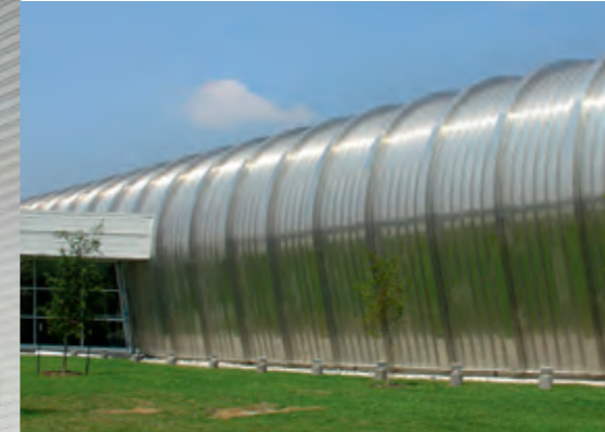
Garland Special Events Center // USA Usage: sports Profile: N65 - 400 Material: 1.0 mm aluminum Color/Surface: bare aluminum Area: 22 300 m²
