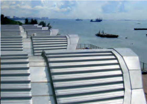
❖ Clifford Pier // Singapore Usage: harbor pier Profile: N65 - 400 Material: 1.0 mm aluminum Color/Surface: silver metallic / PVDF Area: 3 000 m²
