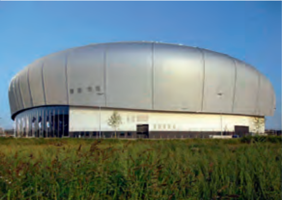
❖ ISS Dome // Germany Usage: sports Profile: BEMO-MONRO® Material: 1.0 mm aluminum Color/Surface: silver metallic / PE Area: 8 000 m²
