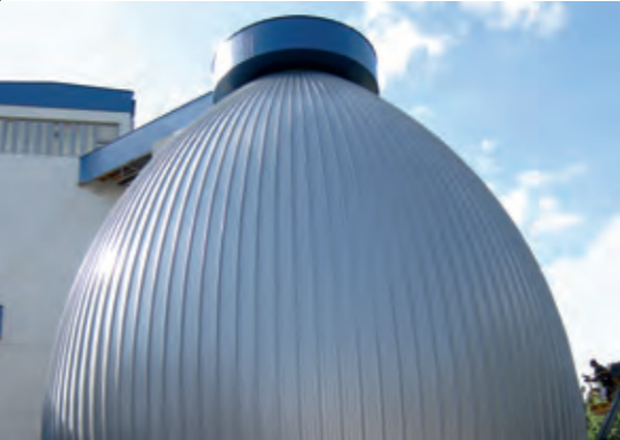
❖ Digestion Tower // Austria Usage: purification plant Profile: BEMO-MONRO® Material: 1.0 mm aluminum Color/Surface: silver metallic / PE Area: 1 000 m²
