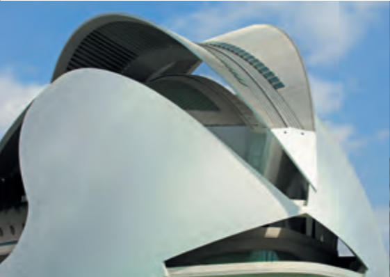
Valencia Opera House // Spain Usage: culture Profile: N65 - 400 Material: 1.0 mm aluminum Color/Surface: stucco Area: 3 600 m²
