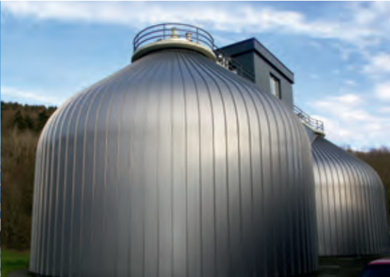
❖ Digestion Tower // Germany Usage: purification plant Profile: BEMO-MONRO® Material: 1.2 mm aluminum Color/Surface: grey metallic / BEMO-FLON Area: 850 m²
