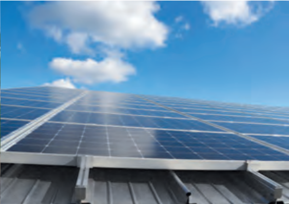
❖ Solar Roof // Germany Usage: industry Profile: VF65 - 422, BEMO-AKKORD Material: 0.8 mm aluminum Color/Surface: stucco Area: 6 400 m²
