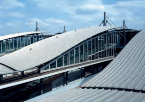
Railway Station // Germany Usage: infrastructure Profile: N65 - 333 Material: 1.0 mm aluminum Color/Surface: stucco Area: 6 000 m²
