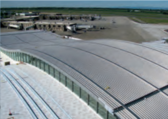
Sacramento International // USA Usage: airport Profile: N65 - 400 Material: 0.85 mm stainless steel Color/Surface: III C Area: 19 000 m²
